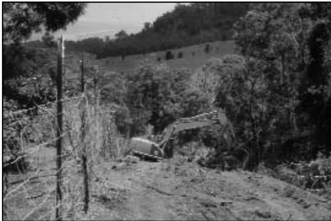
A 30-foot swath was cleared from both sides of the property fenceline to protect new fence from falling trees.
