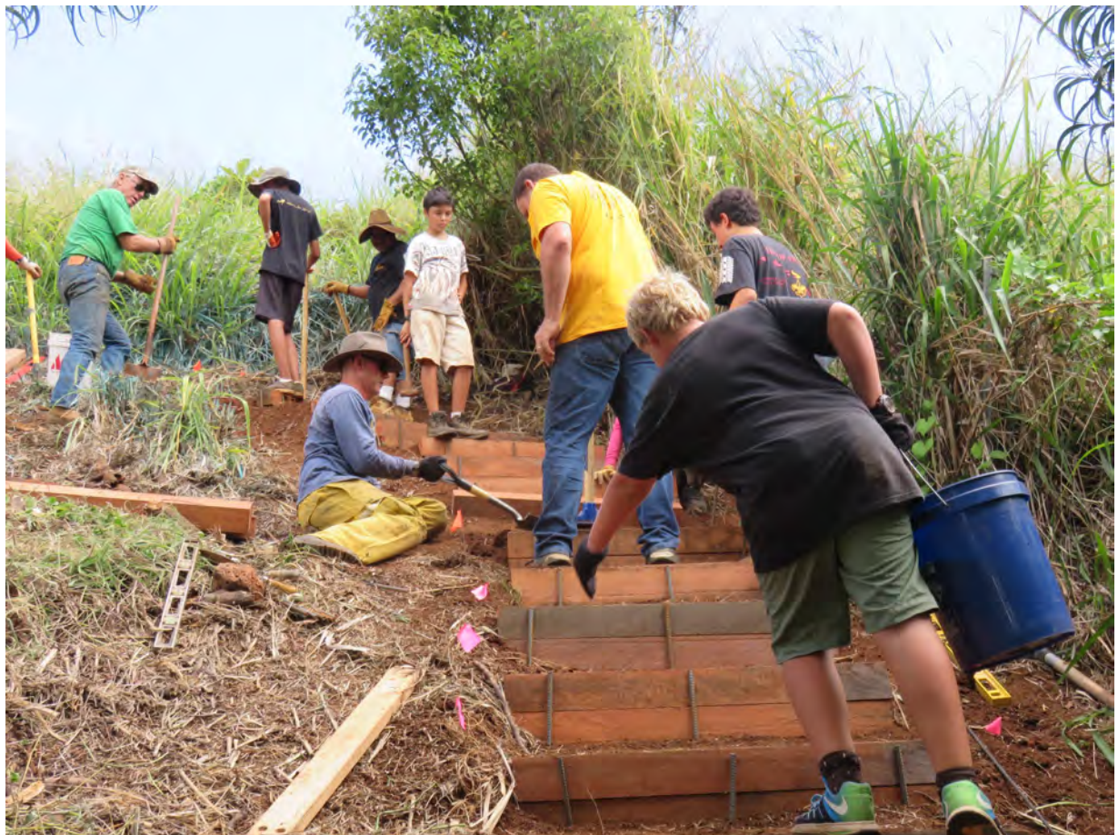
Working as a team, Troop 100 volunteers excavate soil, while widening the trail at base of new steps and haul buckets of soil to use as fill.
