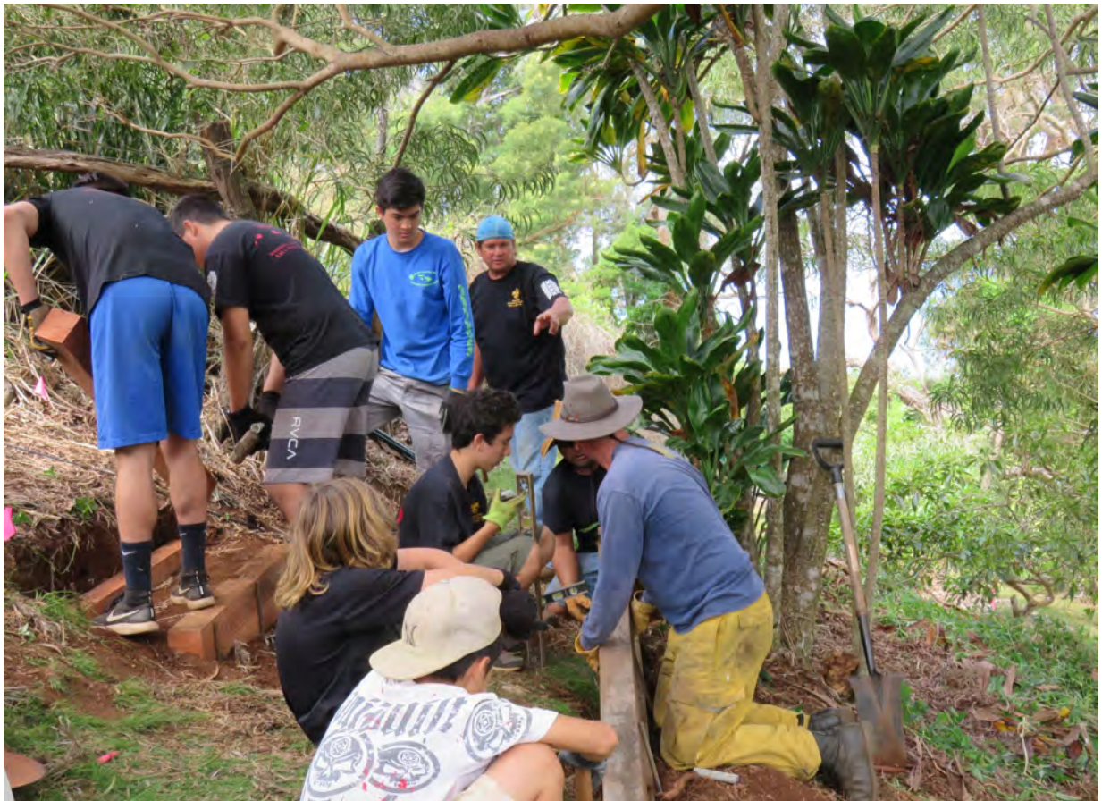
Aolama Chow teaches his crew of 35 volunteers, Scouts of Troop 100, to build steps with proper rise, depth and width. Built into the ground, soil compaction is also important.
